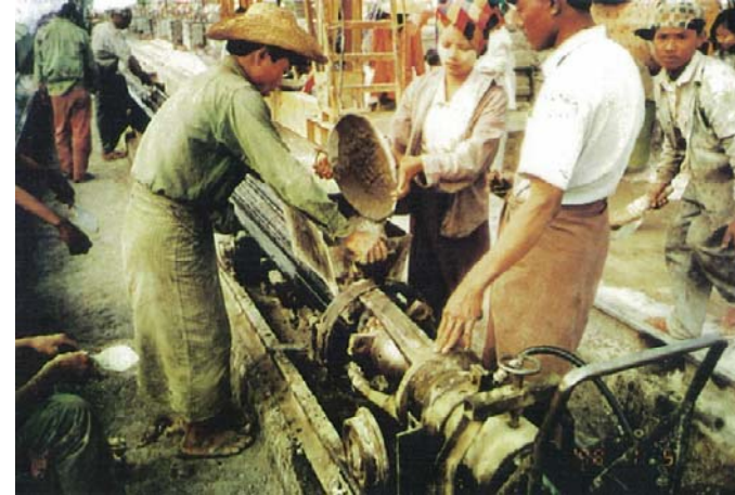
Concrete Pile Production
