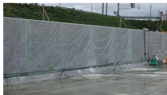
Picture 1 View of Water Supply Curing System.
