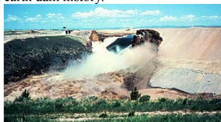
**Fig.1** Breaching of Teton dam
